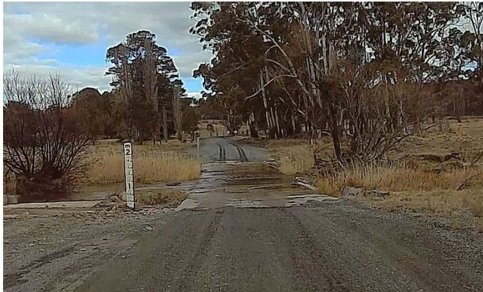
FIGURE 6.3: Looking south from causeway at sealed section of Larbert Rd
