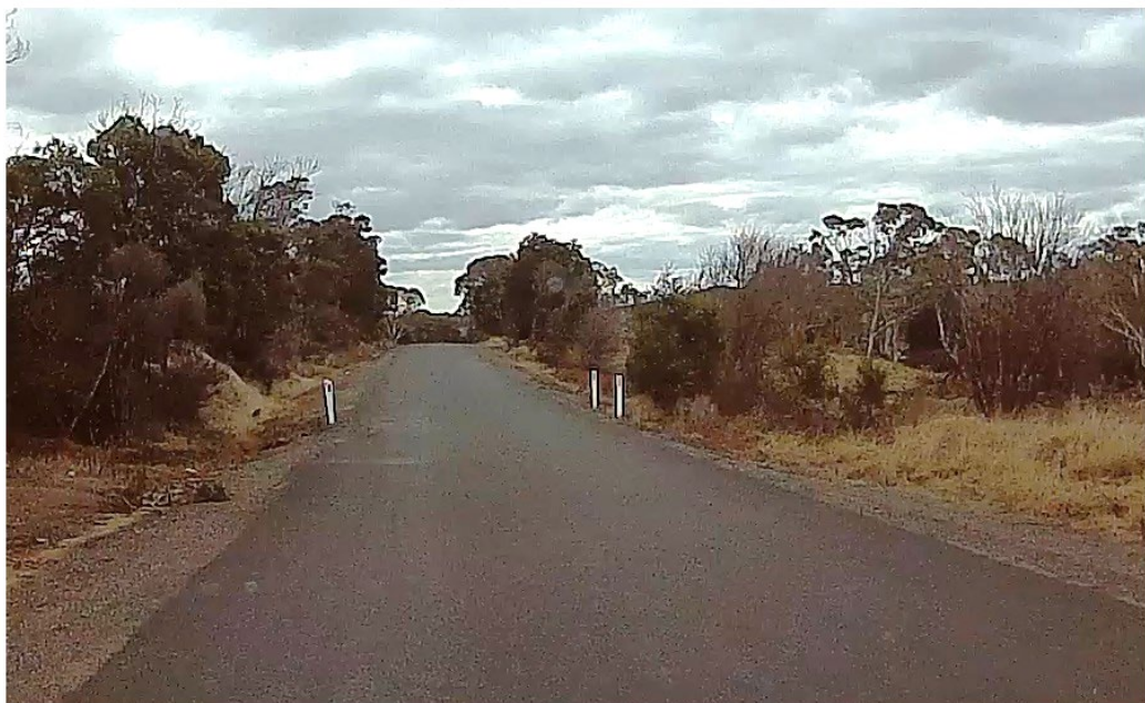
FIGURE 2.2 Typical view of sealed section of Larbert Road
