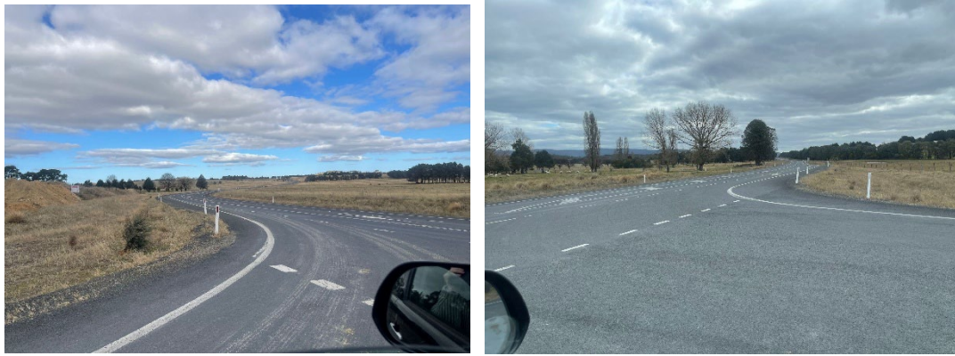
FIGURE 2.5 Sight distance at The Kings Highway from Larbert Road
